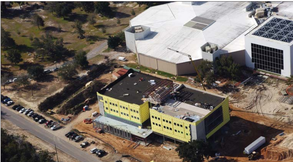
Overhead view of National Flight Academy (under construction) — March 2010.
